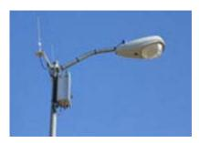
The data collector unit (DCU), in turn, collects meter reads from many meters and securely transmits the gas usage data over a secure wireless network back to PG&E. The DCU shown here is attached to a streetlight.
