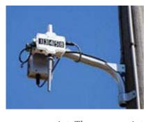
The electric network access point collects meter data from nearby electric meters and periodically transfers this data to PG&E via a secure cellular network. Each RF mesh-enabled device (meters, relays) is connected to several other mesh-enabled devices, which function as signal repeaters, relaying the data to
